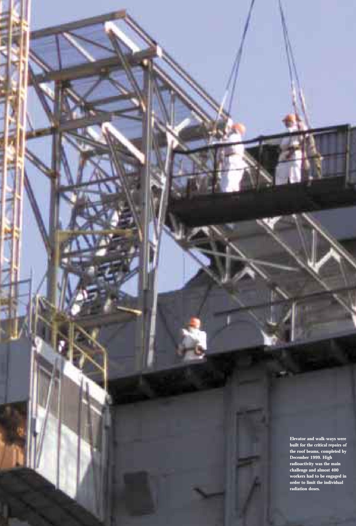
Elevator and walk-ways were built for the critical repairs of the roof beams, completed by December 1999. High radioactivity was the main challenge and almost 400 workers had to be engaged in order to limit the individual radiation doses.
